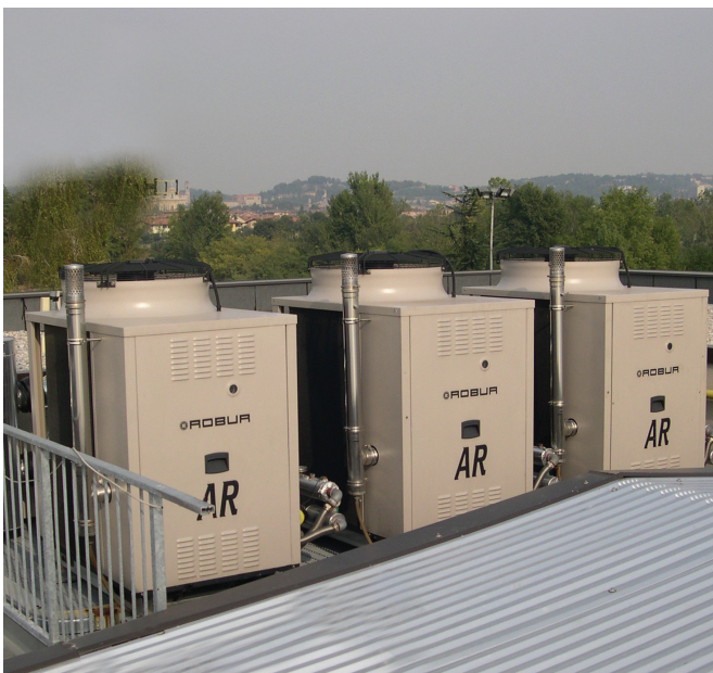
Fig.1 - Front view of Robur GAHP-AR gas absorption heat pumps.
